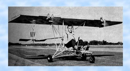
Wilbur Staib built this small airplane in limited hangar space. Two 10 hp West Bend 820 chain-saw engines. Net weight 175 lbs.
