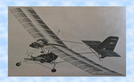
Designed by Ian Becker and Walt Todhunter. Single-seat, high-wing monoplane with 3-Axis control. Empty weight 248 lbs. Structural limits +6 Gs and -4 Gs.
