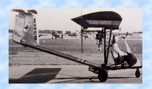
Designed by Marvin Greenwood. Easily transportable. 22 hp engine. Cruise speed 50 mph, stalling speed 26 mph. Structural limits +3.8 Gs and -2 Gs.
