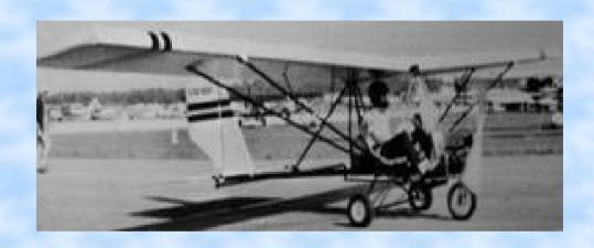
Low front mounted engine with tricycle landing gear and strut braced double surface wing. 3-axis control.
