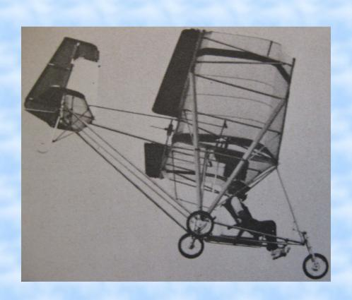
Designed by Nile Downer. Aluminum alloy tube airframe. Empty weight 243 lbs. Payload 257 lbs. Cruise speed 40 mph and stall speed 22 mph. Climb rate 650 fpm.
